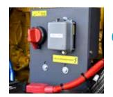
**Safety First** The battery cutoff switch and external emergency stop provides additional safety.
