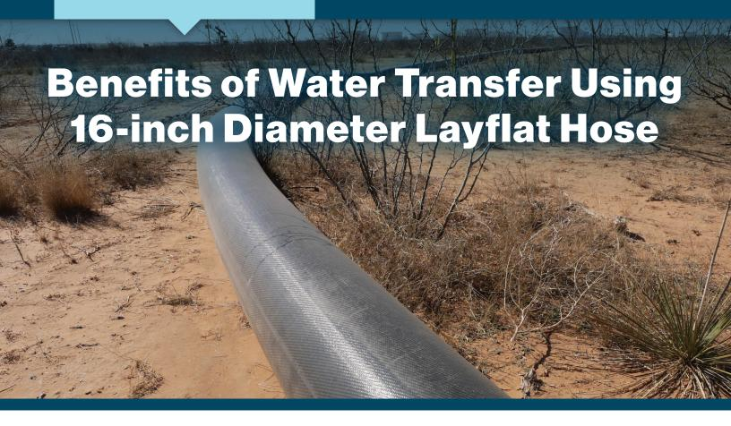
A smarter way to transfer water over distance can be the use of **16-inch layflat hose** instead of 12-inch systems. 16-inch systems reduce head pressure and save on fuel consumption and, in some instances, can eliminate the need for two 12-inch pipelines. Contact us to learn more.
